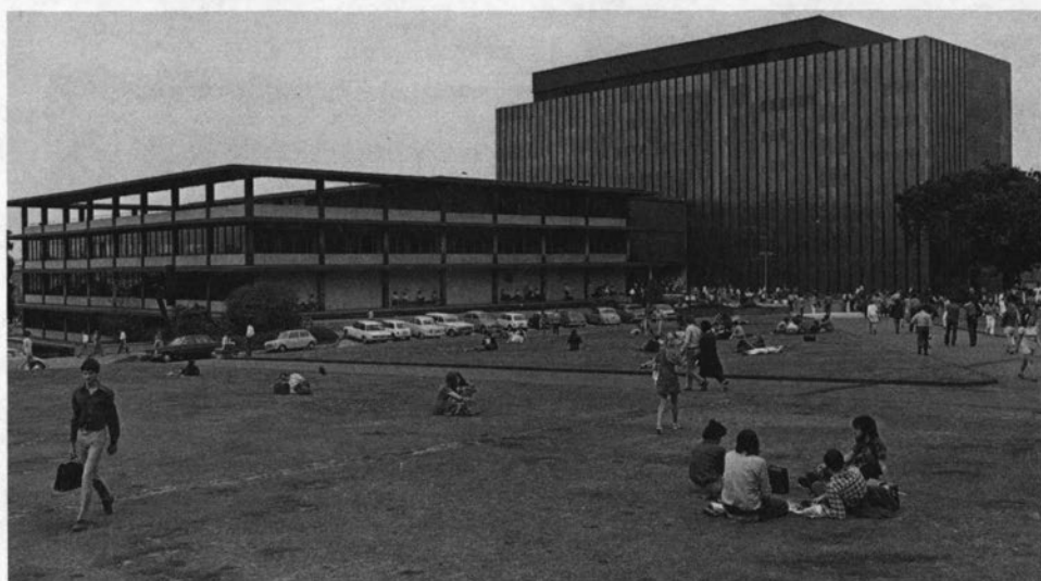
Fisher Library, University of Sydney. Designed by T. E. O'Mahoney and the state government architect of N.S.W., Fisher, Australia's largest and heaviest used academic library building, was erected in two stages, 1963-1971. It grosses 23,225 square meters and provides space for 3,100 readers and three million volumes.
