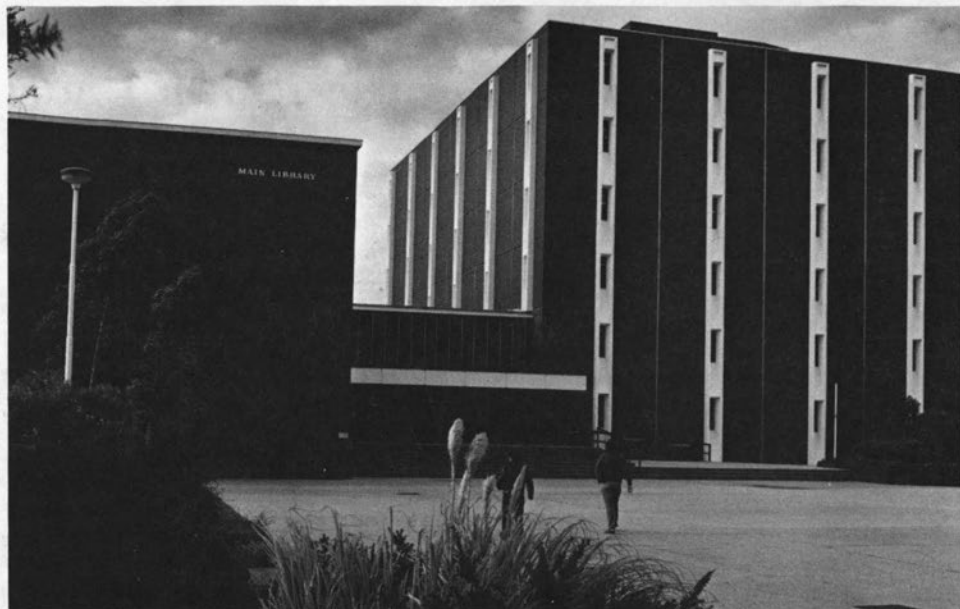
Monash University Main Library. This building, erected in three stages, 1964–1974, has accommodation for 816,000 volumes and 2,113 readers. It is complemented by three separate and reasonably adjacent buildings housing collections and services respectively in law, biomedical sciences, and applied sciences and engineering.
