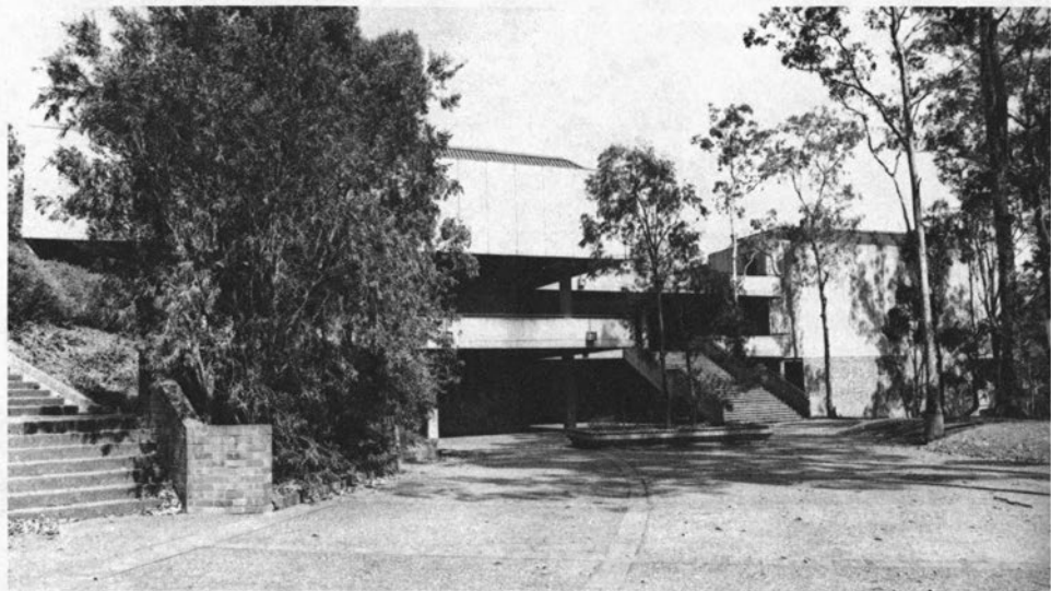
Auchmuty Library, University of Newcastle. The first two stages of a planned three-stage building, this library houses 300,000 volumes and 1,000 readers. Campus planners have made a conscious effort to retain the Australian eucalyptuses that clothe the site.
